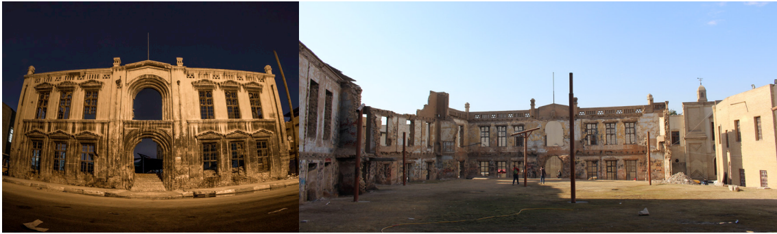
Photos of the remaining facade
